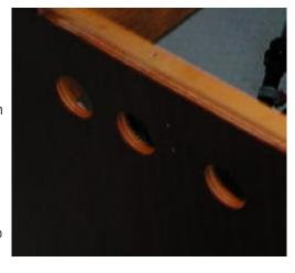
9. Install the box in the pantry cupboard and fix to the three enclosed sides and at the bunk side by the two wooden blocks at the sink partition and cupboard partition under the sink bowl. If the box is placed at the correct height then a light pressure is obtained from the sink top which compresses the box slightly helping to keep it fixed. Finish the box's upper edge with joined PVC edging 50 x 50mm and glue with Sikaflex.
