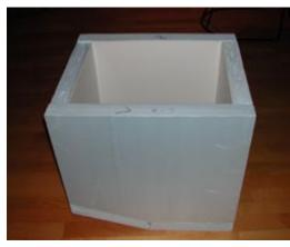
the exact inner dimensions of the foam construction. (Mark with a Stanley knife and break along the cut line). Apply tile glue with a glue spreader, place the PVC sheet and press firmly. After drying, seal with Sikaflex and smooth with a wet soapy finger.
