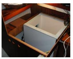
12V. Fix the remote control and cold air supply hose with a hoseclip to the fan. Make sure you lead this through the cut-out under the bunk. Place the armature in the cut out and fix with the bolts. Now you can see the reason of the glued nylock nuts. Remove the old ledges from the lid under the cupboard top. Fit the cupboard top and other disassembled wooden parts. The fixed part is now ready.
